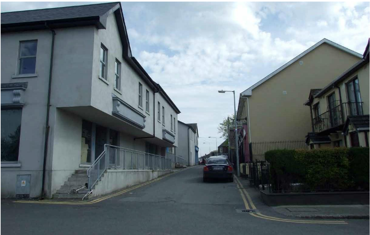
Disconnected retail unit and street along Fagan's Lane
