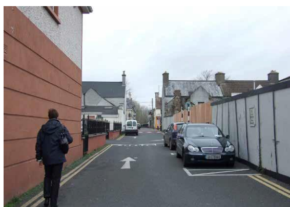
View of Doctors Lane showing poor street frontage, poor public realm and vacant site
