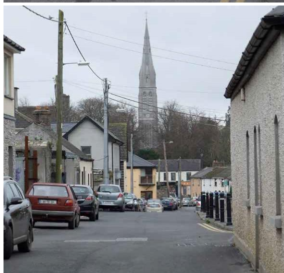
Poor definition of the public realm along Pound Lane
